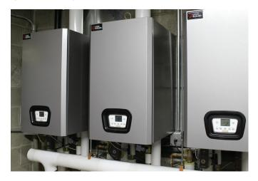
Because of the size limitations in the mechanical room, the existing equipment had to be removed before the new boilers could be installed (supplemental space heaters were used to maintain the temperature required for the reptiles in the exhibits).
