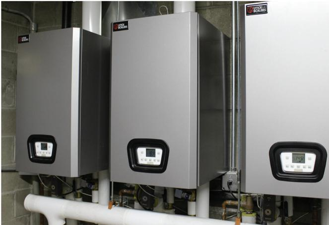
Because of the size limitations in the mechanical room, the existing equipment had to be removed before the new boilers could be installed (supplemental space heaters were used to maintain the temperature required for the reptiles in the exhibits).
