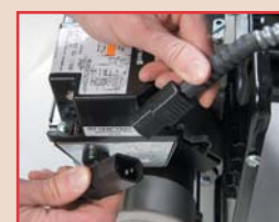
Beckett burner with plug 'n play connector
