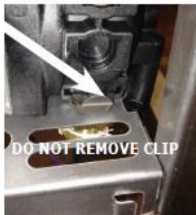
RIGHT SIDE CLIP - INSIDE BOILER JACKET
