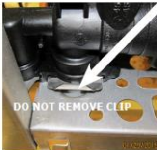
LEFT SIDE CLIP - INSIDE BOILER JACKET
