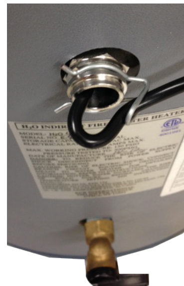
Figure 3 - Sensor Wire Secured to Well With Clip
