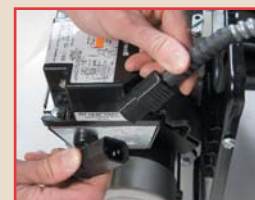
Beckett burner with plug 'n play connector
