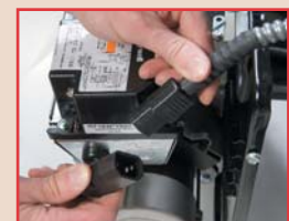
Beckett burner with plug 'n play connector
